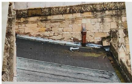
outh nave aisle roof east abutment with south transept west wall – lead flashing has been damaged & torn (possibly due Tempted theft); felt in very poor condition; stonework poorly course, open jointed and roughly patched with cement mort
